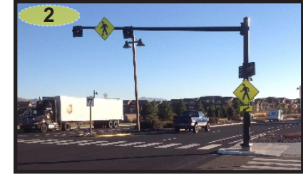
Existing pedestrian activated flashing system.
