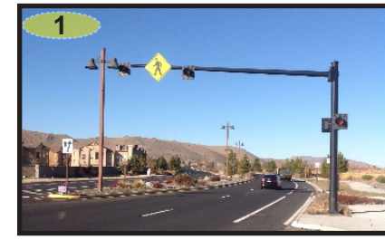
Existing pedestrian activated flashing system.
