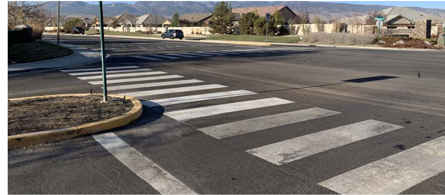
Pedestrian Crossing and Safety
