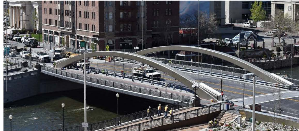
VIEW OF BRIDGE
