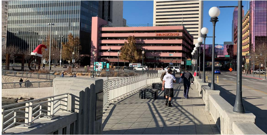
CENTER STREET BRIDGE DOUBLE RAILING
