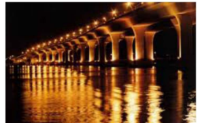
UNDER BRIDGE LIGHTING
