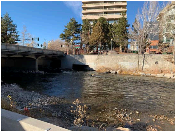
EXISTING FLOOD WALL
