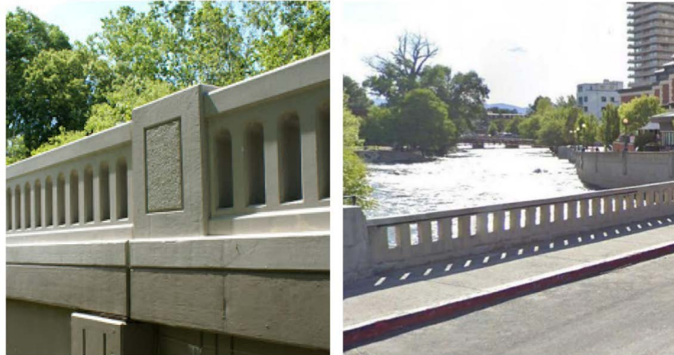
OPEN DECORATIVE CONCRETE VEHICULAR GUARDRAIL
