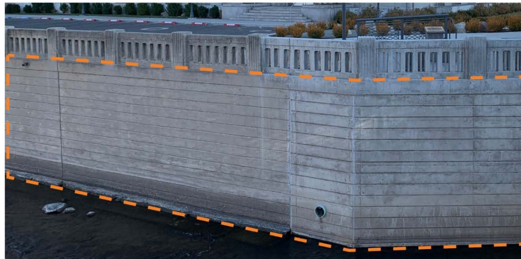
FORMLINER PATTERN FOR FLOOD WALL
