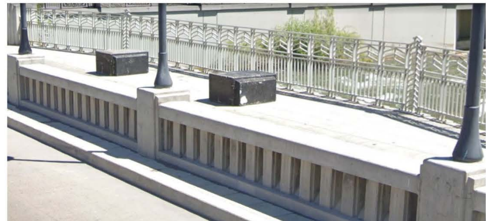
DECORATIVE RAILING AND GUARDRAIL
