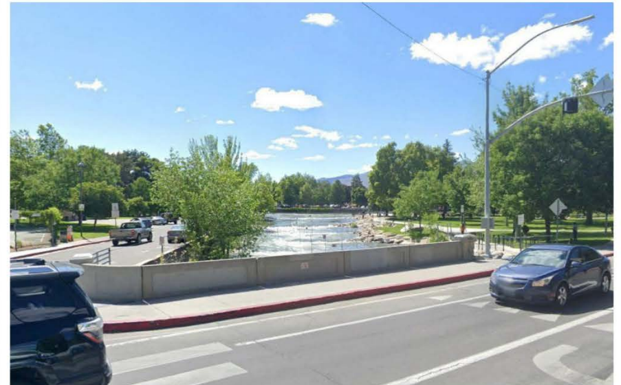
SOUTHERN BRIDGE SECTION, LOOKING WEST
