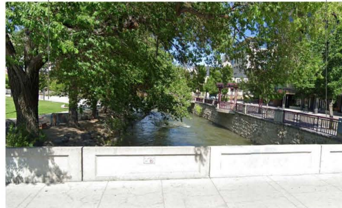
SOUTHERN BRIDGE SECTION, LOOKING EAST
