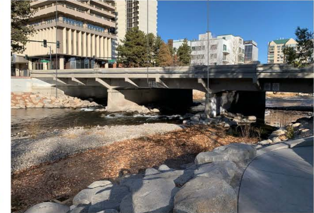
VIEW OF NORTHERN BRIDGE
