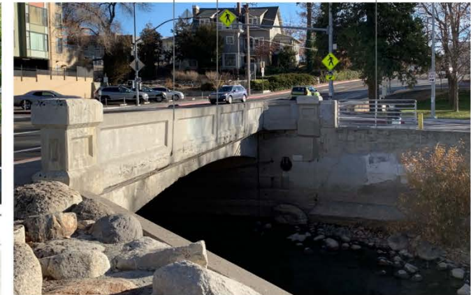
VIEW OF SOUTHERN BRIDGE
