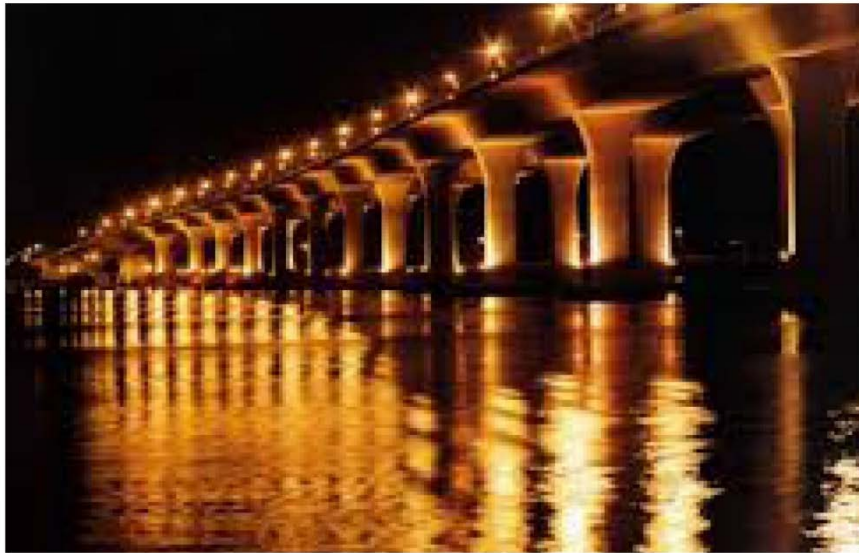
UNDER BRIDGE LIGHTING
