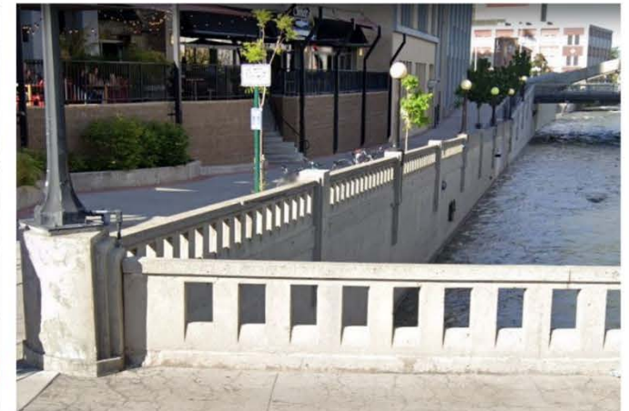
OPEN DECORATIVE CONCRETE RAILING
