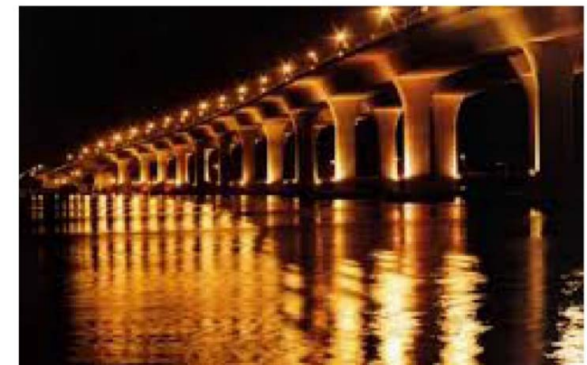
UNDER BRIDGE LIGHTING
