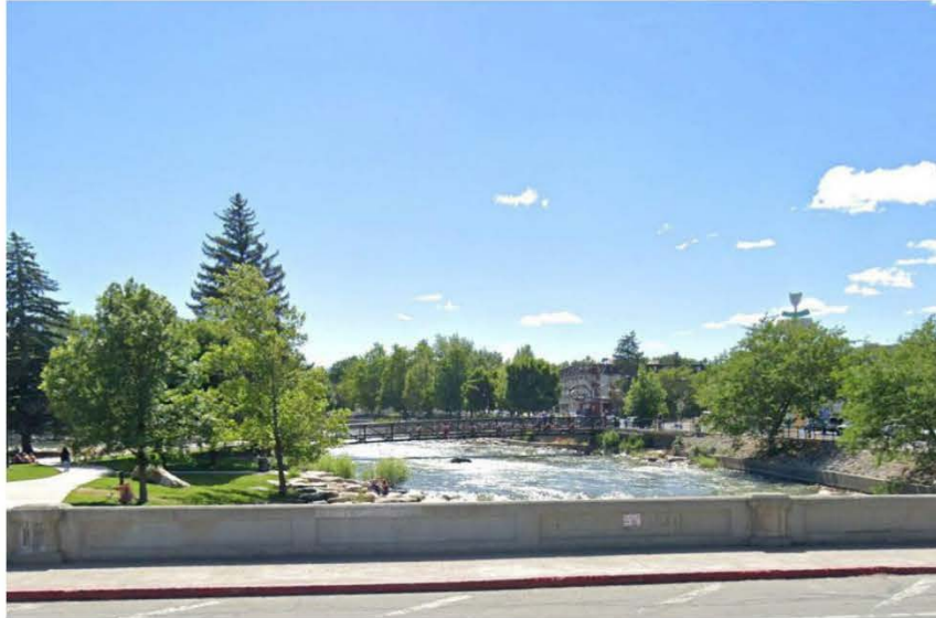
NORTHERN BRIDGE SECTION, LOOKING WEST
