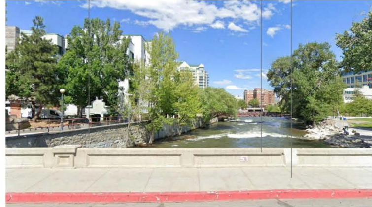
NORTHERN BRIDGE SECTION, LOOKING EAST
