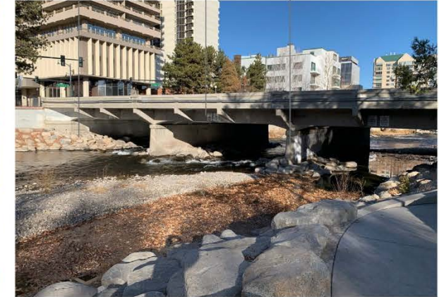
VIEW OF NORTHERN BRIDGE
