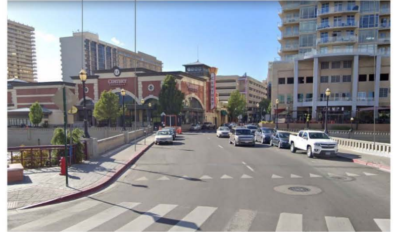
VIEW LOOKING NORTH
