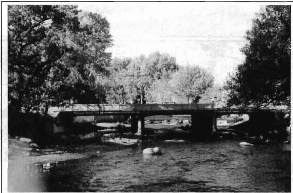
Photograph 1: North Arlington Avenue Bridge, east side, camera facing west, 10/26/01.
