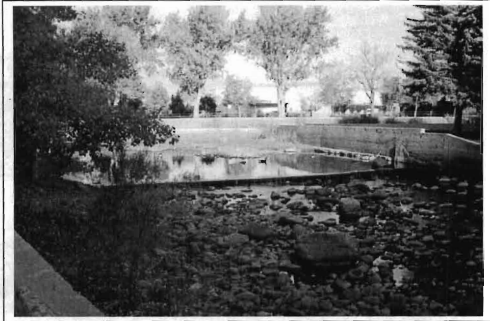
Photograph 3: Wingfield Park Dam, south side, camera facing northwest., 10/26/01.
