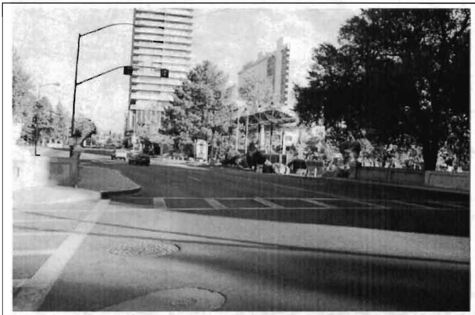
Photograph 2: South Arlington Avenue Bridge deck, camera facing north., 10/26/01
