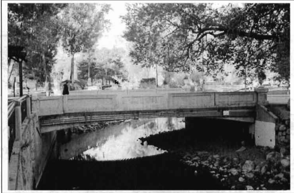
Photograph 1: South Arlington Avenue Bridge, east side, camera facing west, 10/26/01
