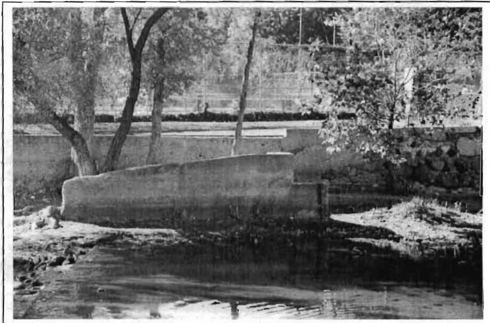
Photograph 4: Wingfield Park Dam, south side fish ladder, camera facing southwest, 10/26/01.
