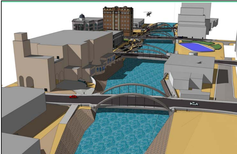
Bridge Supported from above with Tied Arch
