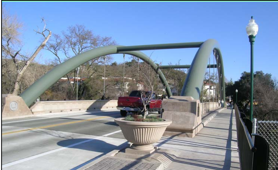
Above Supported Bridge Tied Arch Bridge in Atascadero, CA
