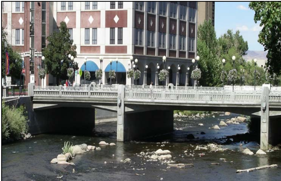
Below Supported Bridge - Center St
