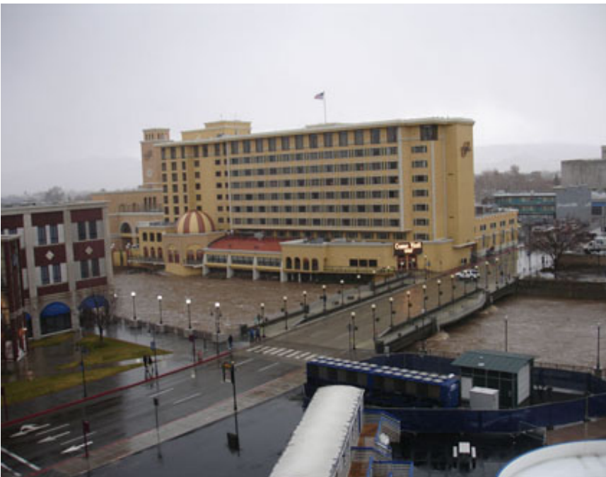
Looking Southeast at Sienna Hotel from Cal Neva Garage
