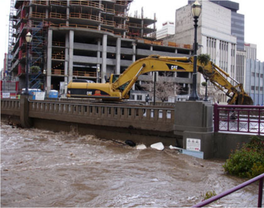
Looking Northeast at upstream side of Sierra
