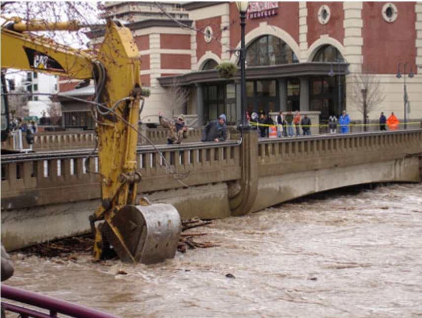
Looking upstream at South Span of Sierra Street
