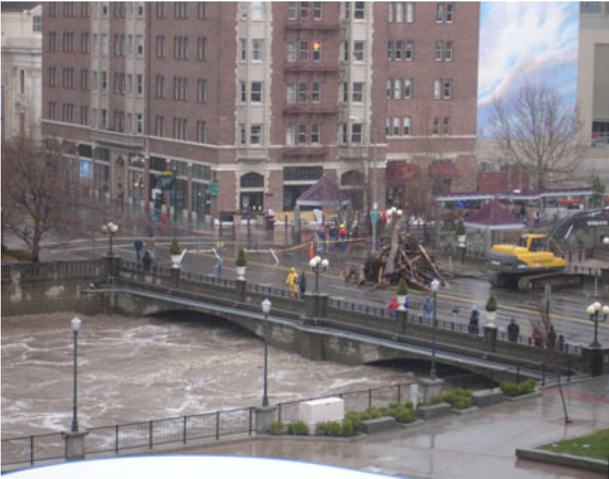
Looking Southwest (at downstream side) at Virginia Street from Cal Neva Garage
