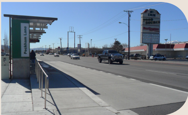
Figure 5.5 - Bus Lane in Virginia Street
