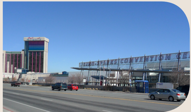
Figure 5.3 - Roadway width not safe for uncontrolled pedestrian crossing
