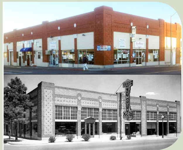
Figure 4.1 - Old brick structure used for businesses (pictures courtesy of Barry O'Sullivan)
