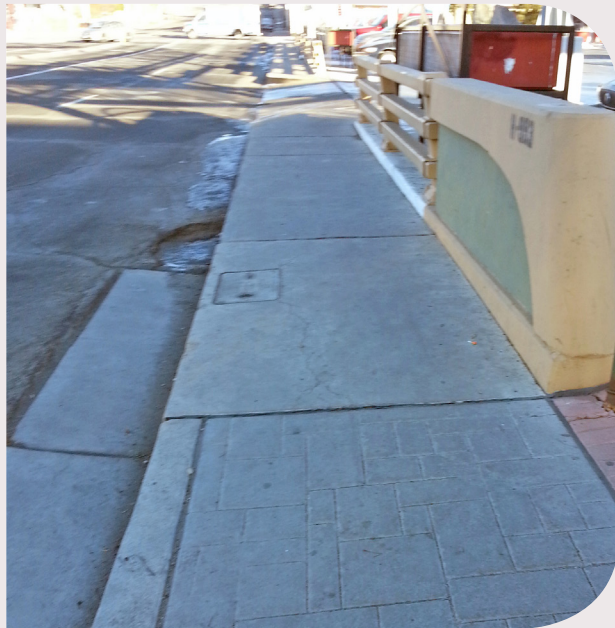
Figure 2.6 - Narrow sidewalk at the bridge crossing I-80
