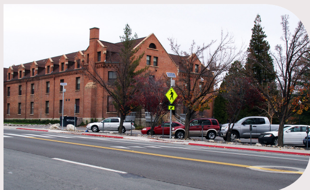
Figure 2.1 - University of Nevada, Reno. Manzanita Hall
