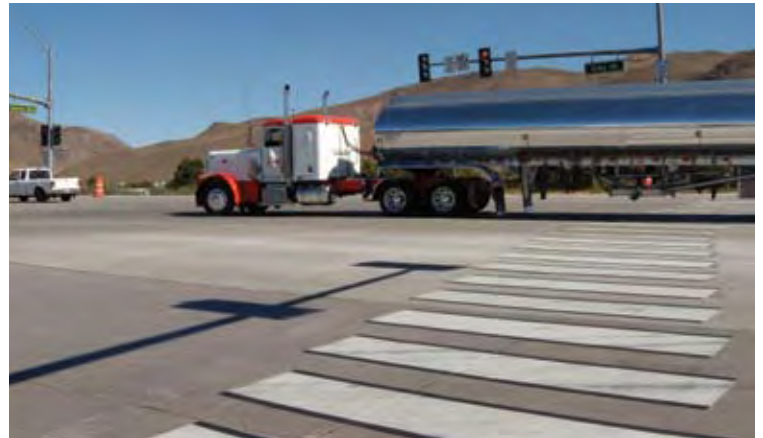
Back in Business — Greg Street is back in business now that reconstruction efforts finished five weeks early. The intersection of Greg Street and Sparks Boulevard, a major travel point for warehouse distribution with high truck traffic, is reopened with a new surface especially designed for durability. Design consultants PBS&J, of Reno and contractors Q&D Construction, of Sparks, partnered with RTC Project Manager Garth Oksol on the $5 million project. Work included new concrete paving on Greg Street from Sparks Boulevard east to Vista Boulevard which is designed to withstand high volumes of heavy loads over a long lifespan.
