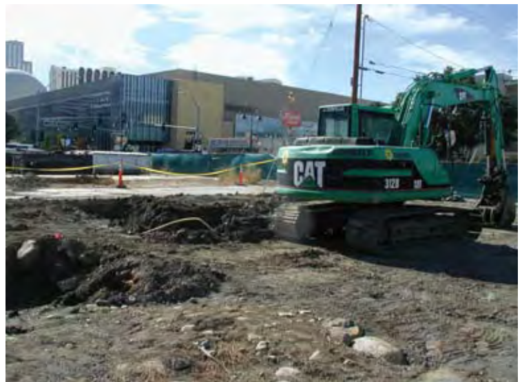
Crews begin site preparation for RTC 4TH STREET STATION.
